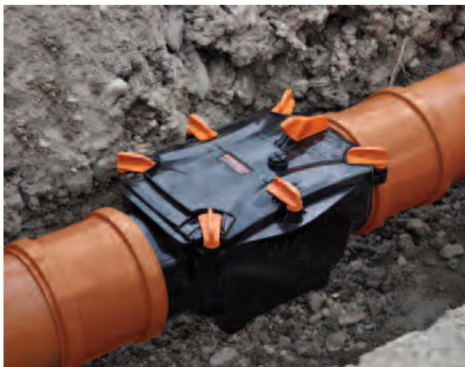
Installazione a vista / Installation at sight
